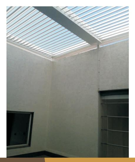
The louvers are operated by a hand-held remote. Open the louvers slightly to increase ventilation, or a full 180 degree allowing maximum sunlight into your Jacuzzi. Your new Jacuzzi roof has the stylish look and feel of a traditional pergola with the benefits of a fully adjustable louvered system. Having toughened glass along with D'cent Roof Louvers allow you to get the natural light 24/7 and ventilation with the louvers
